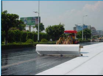
Geotextile in highway
