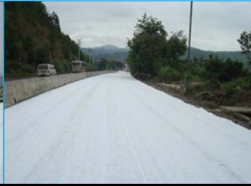
Geotextile in road
