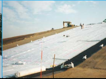
Geotextile liners in slope
